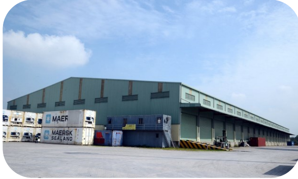
CFS & BONDED WAREHOUSE
